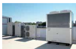
2012 New GHP units. Panasonic's gas-driven VRF Systems are ideal for projects where power restrictions apply.
